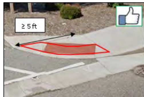
Solution 2. DWS should be in a radial pattern beyond the ramp when the bottom of the ramp is greater than or equal to 5 ft from the back of curb.
